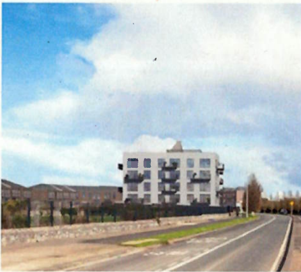
View of Block 1 on approach to Site
